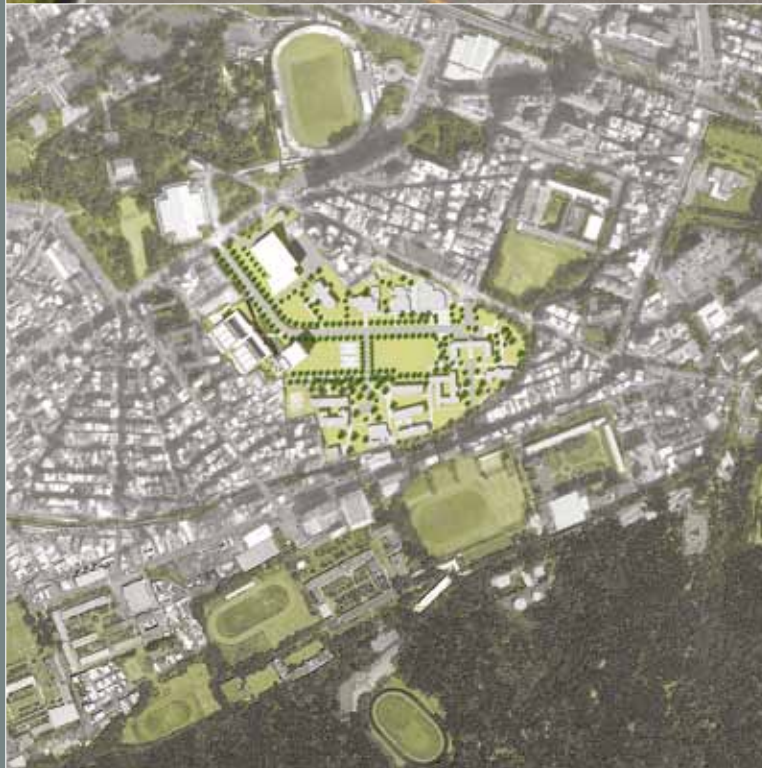
National Chiao Tung University (NTCU), Bio-Tech Building Credits: Leers Weinzapfel Associates
